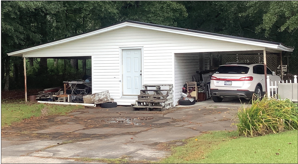
A. Circa-1980 Carport and Storage Shed Oblique View, Facing Northeast
