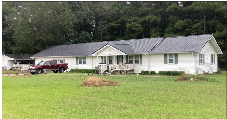
B. Oblique, Facing North-east
