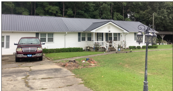
D. Façade Detail, Facing Southeast
