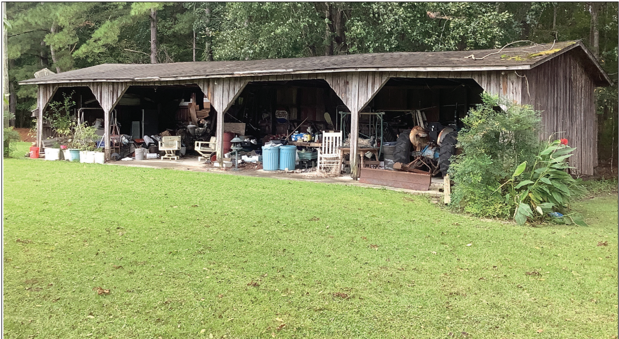
B. Circa 1980 Partially Enclosed Shed Building Oblique View, Facing Northeast
